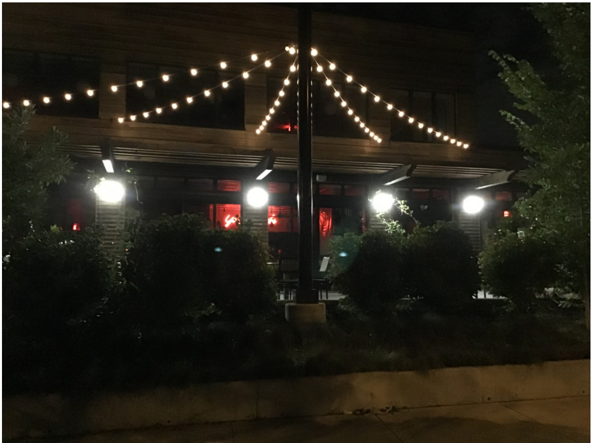
Unshielded perimeter lighting - glare and light trespass
